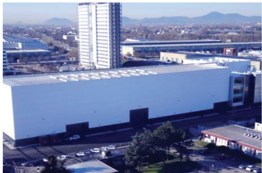
Fig. 5 Neutral Beam Test Facility in Padua, Italy Source: courtesy of Consorzio RFX
