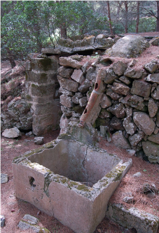
FIGURE 11 Ruins of an ancient roof-and-tank set
