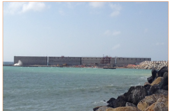
FIGURE 10 4 REWEC3 caissons completed up to 10m above M.W.L. at the Port of Civitavecchia (Rome, Italy)
