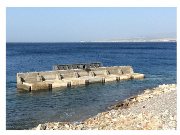
FIGURE 1 The REWEC3 plant installed in the breakwater in reinforce concrete at NOEL laboratory
