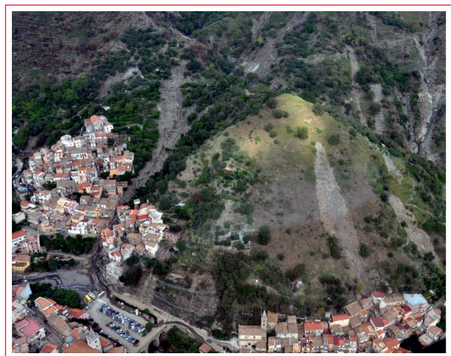
FIGURE 1 Some debris-mud flows occurred in the area on October 1 st , 2009
