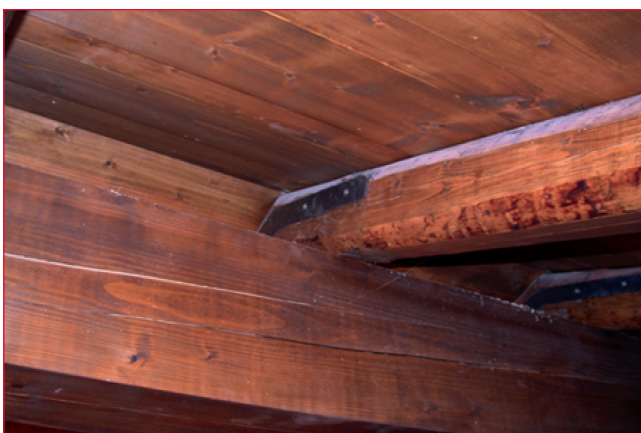
FIGURE 34 Metal connections to roof elements
