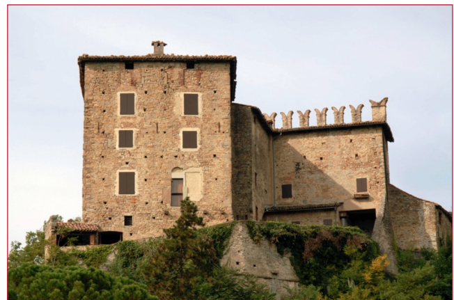
FIGURE 8 General view from south-east
