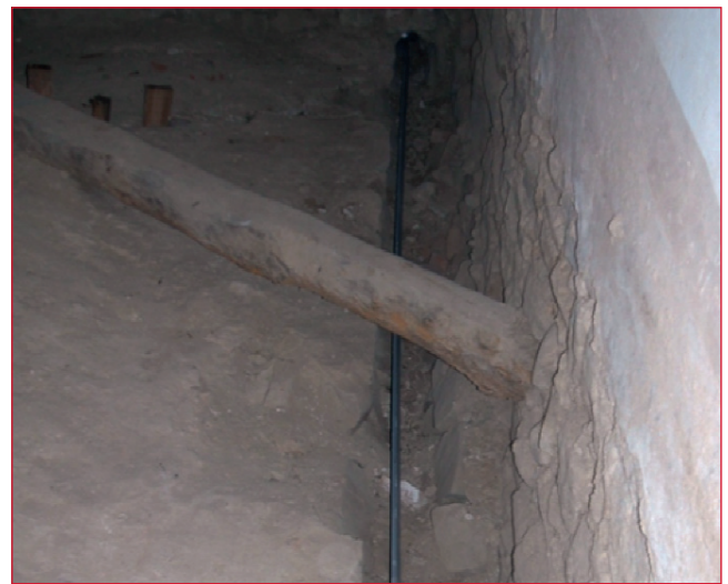
FIGURE 31 Steel tie-rod at the extrados of vault
