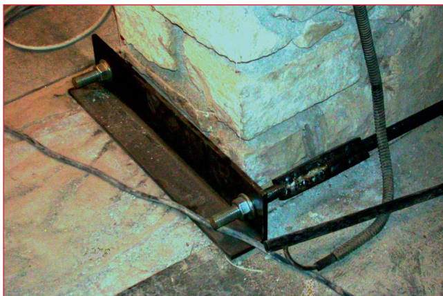
FIGURE 32 Example of internal tie-rod anchorage
