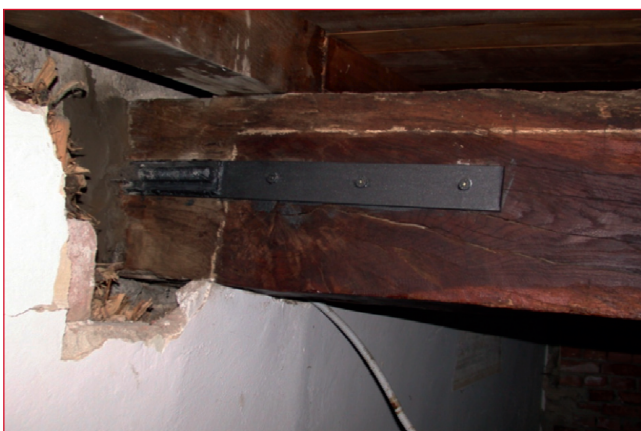
FIGURE 33 Connection floor-wall
