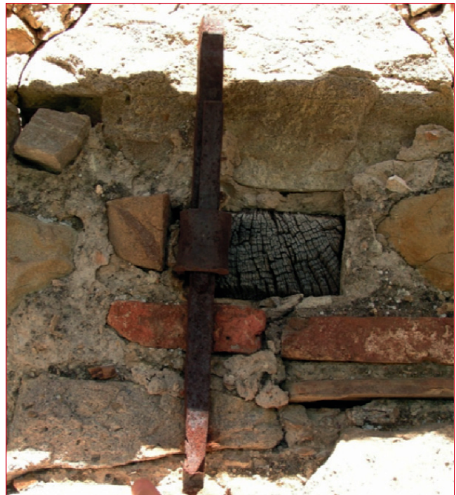
FIGURE 26 Wooden chain with metal anchor
