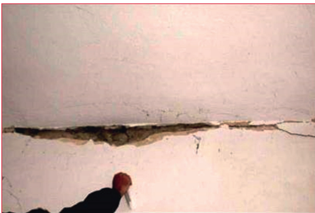
FIGURE 17 Wall-floor detachment
