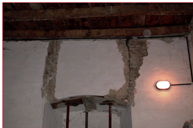
FIGURE 19 Detachment of walled-up window
