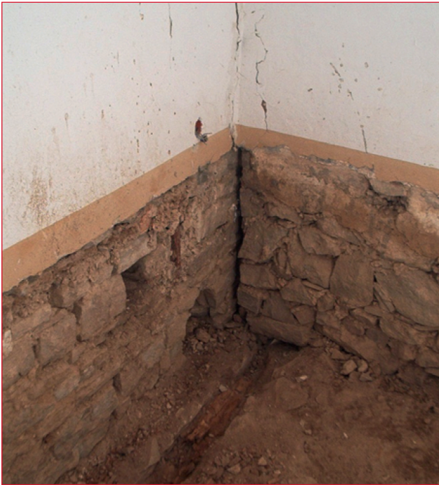
FIGURE 27 Remains of the ancient wooden tie
