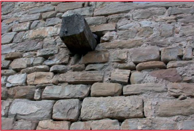
FIGURE 10 Example of masonry texture
