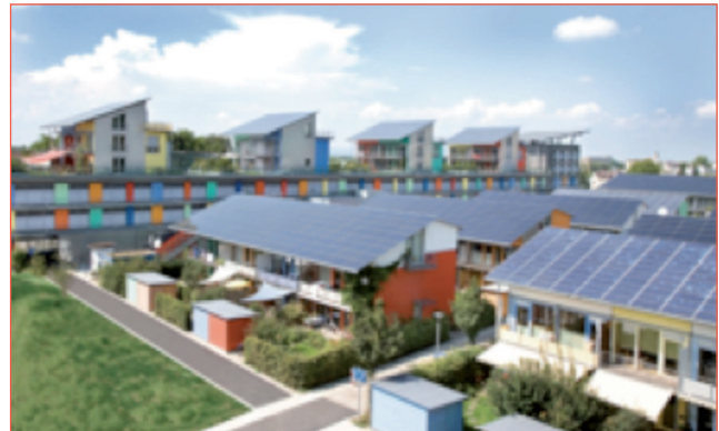
FIGURA 1 Net Zero Energy Buildings Cluster / new settlements. Plus energy settlement in Freiburg (Germany), design: Rolf Disch. The Plus Energy Settlement in Freiburg is an example where the zero energy balance is achieved in the frame of an estate. Some of the 59 built terrace houses have a positive primary energy balance, others a negative one. The average is clearly positive. The efficient row houses are covered with 3150 m 2 of roof top integrated PV generators. The heat is supplied by district heating. The efficiency of the houses bases on the Passive House concept and a consequent (urban) planning for shadow-free south orientation, position and shape of the buildings Source: Rolf Disch
