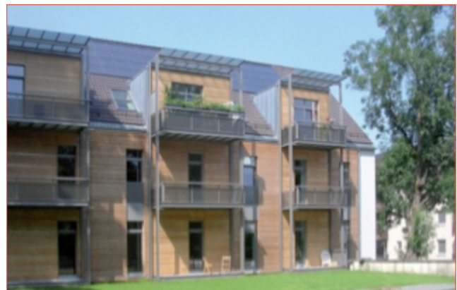
FIGURA 2 Net Zero Energy Buildings Cluster/ retrofit projects. Renovated district in Bad Aibling (Germany), design: Schankula-Architekten. New buildings generate an energy surplus to compensate negative balances of refurbished former military accommodation buildings from the 1930s. ST and PV areas differ significantly from each other. In the shown example, heat is fed into the local heating grid of the settlements by means of 2000 m 2 of ST collectors Source: Schankula-Architekten
