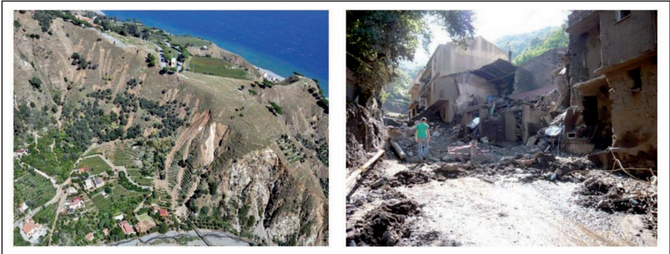
FIGURE 2 Panoramic view of a slope interested by a pervasive series of mud/debris flows in the Briga catchment and damages after the October 1, 2009 event in Briga village
