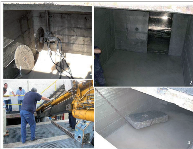
FIGURE 9 Connection sequence for junction of feeding flow splitter chamber and new biological basin
