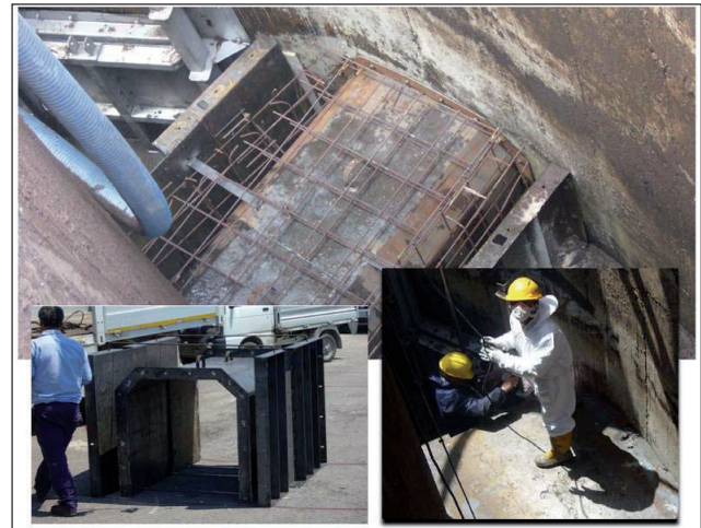
FIGURE 10 Crossing channel of intermediate section in the existing flow splitter
