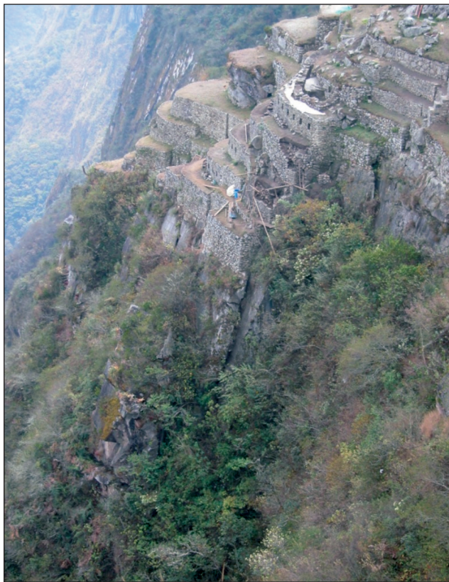
FIGURE 4 Open fractures in the SW flank below the Inca citadel Source: ENEA
