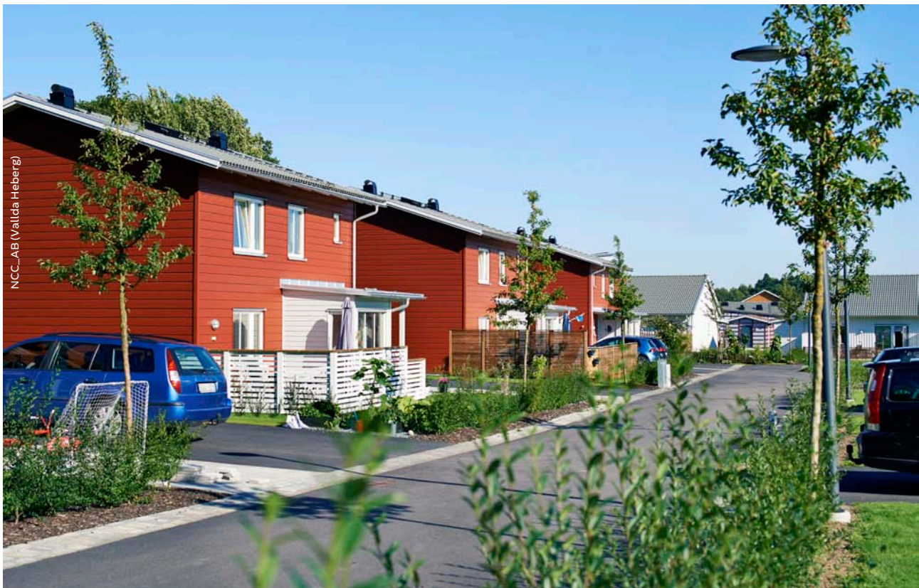
Fig. 4 Sweden: single-family house in Vallda Heberg
