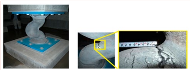
PHOTO 1 Crack on the surface of a lead damper
