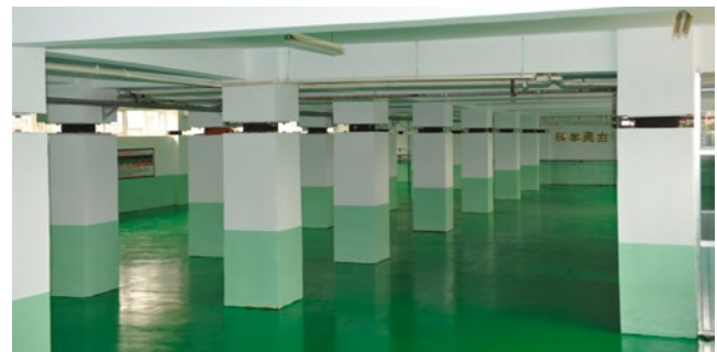
FIGURE 20 Isolation system installed in 1st storey of a retrofitted school
