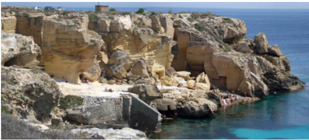
FIGURE 2 Rock blocks fallen at Cala del Bue Marino
