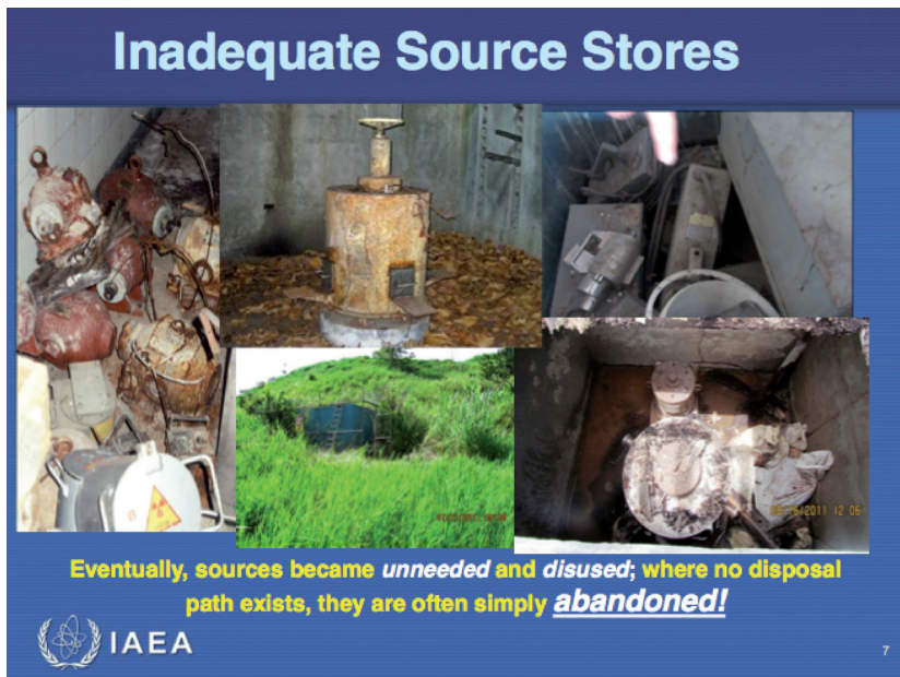
FIGURE 3 Example of inadequate source store Esempi di depositi inadeguati per le sorgenti Source: IAEA, International Conference on the Safety and Security of Radioactive Sources, Abu Dhabi, Oct 2014
