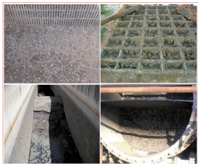
FIGURE 2 Biofouling colonization residual inside cooling water system [1]
