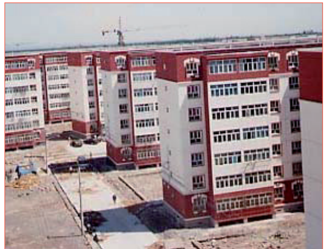
FIGURE 3 Base isolated masonry buildings in China
