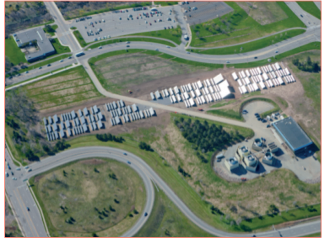
FIGURA 4 On-site energy generation as a part of the landscape design. The Solar Strand, Buffalo University Campus, Buffalo (US), 2011. Design: Walter Hood, Hood Design. The solar array powering the existing dormitory of the Campus. The PV modules on the ground are arranged according to a DNA pattern. They give form to a public space in a direct functional and visual relationship with the buildings of the campus Picture ©2012 University at Buffalo
