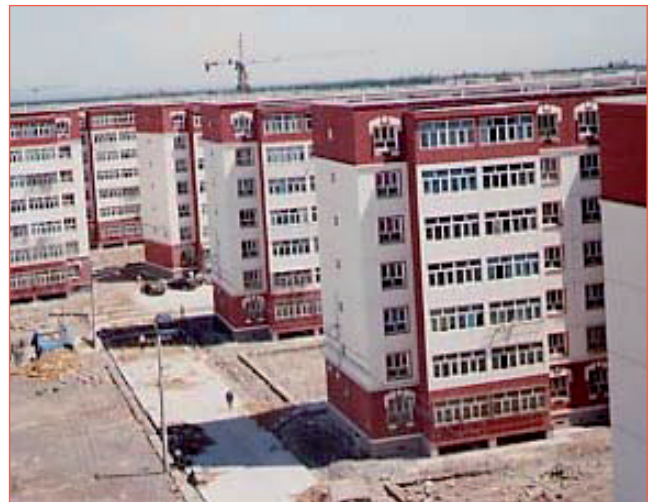
FIGURE 3 Base isolated masonry buildings in China
