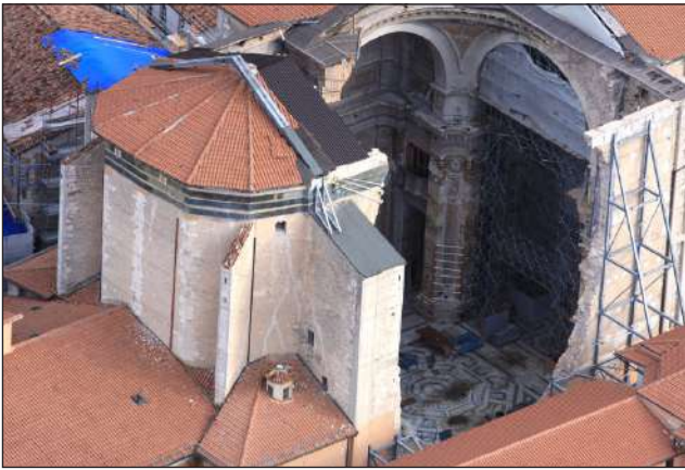
FIGURE 10 Securing the Duomo in L'Aquila, following the 2009 earthquake Source: Author's personal archive
