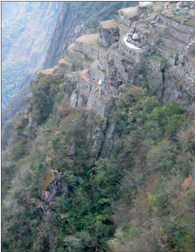
FIGURE 4 Open fractures in the SW flank below the Inca citadel Source: ENEA
