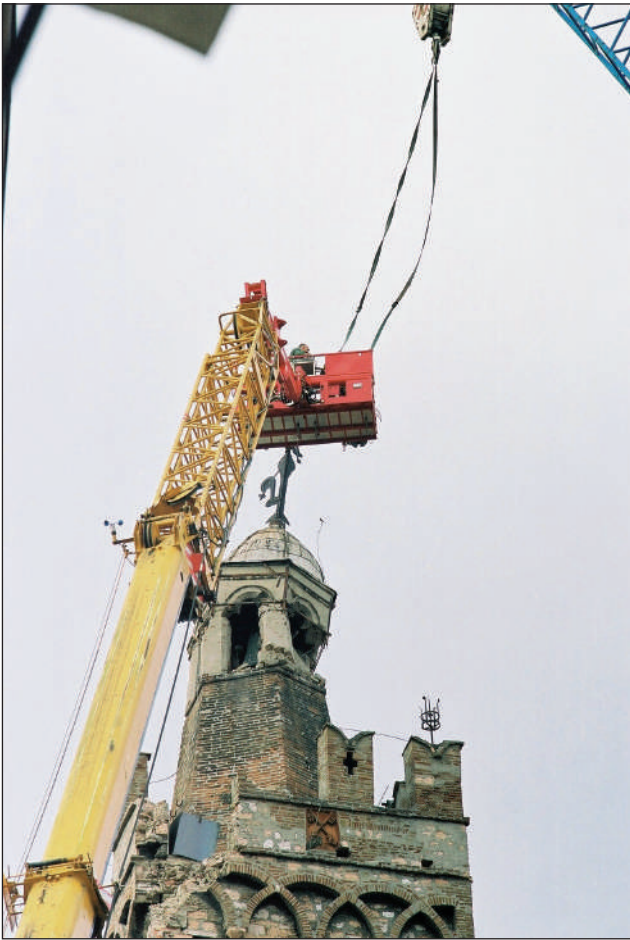
FIGURE 3 Securing the Torrino in Foligno, following the 1997 earthquake Source: Author's personal archive
