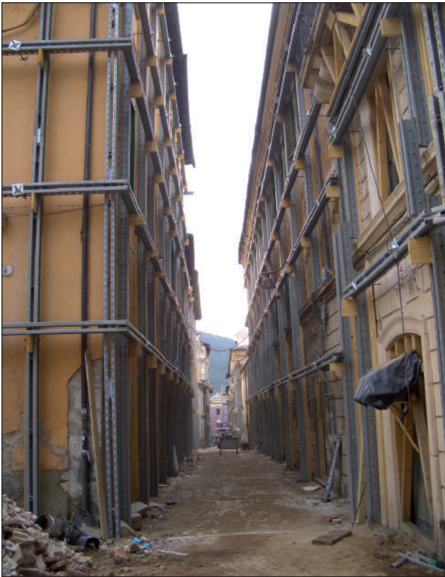
FIGURE 11 Securing historical palaces in the historical centre of L'Aquila, following the 2009 earthquake Source: Author's personal archive
