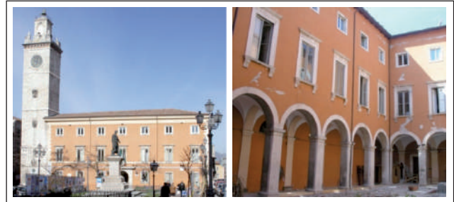
FIGURE 1 Palazzo Margherita: main façade and courtyard Source: ENEA
