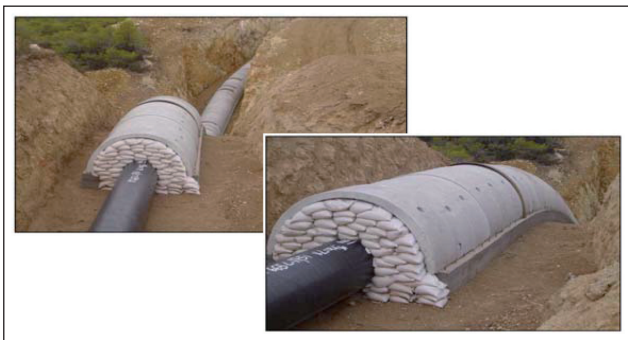
FIGURE 9 Megara to Korinthos High Pressure Natural Gas Pipeline. Encasing of pipeline at active faults crossings Source: http://users.ntua.gr/gbouck/proj-photos/megara.html
