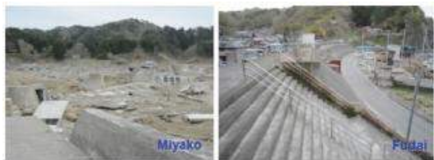
FIGURE 8 a) Protective wall in Miyako destroyed by the tsunami; b) Protective wall in Fudai
